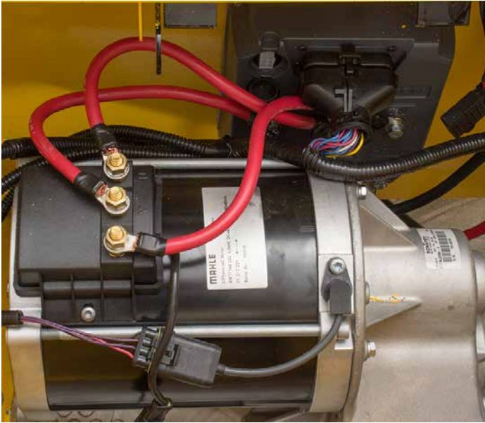
Figure 14: The motor connected to the Sevcon motor controller.
